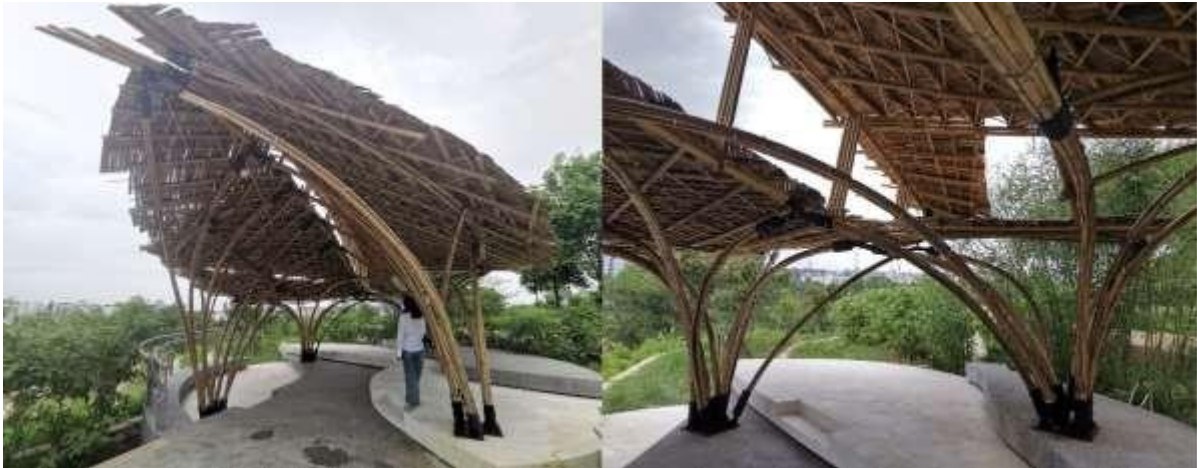
Fig. 18. Experiment of Bamboo pavilion using multiple connectors in one node at bases by Thammasat Bamboo studio.
