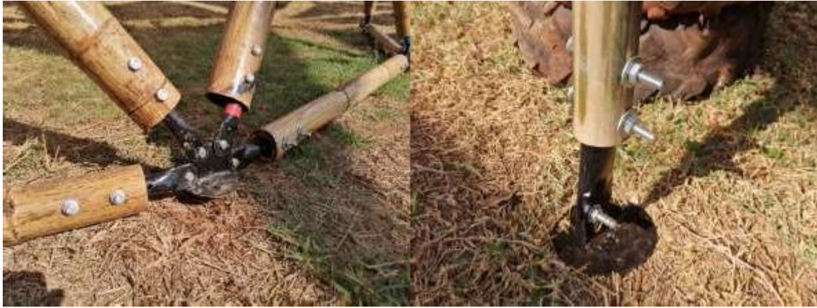
Fig. 14. Star plates that are designed to connect super structure to the ground.
