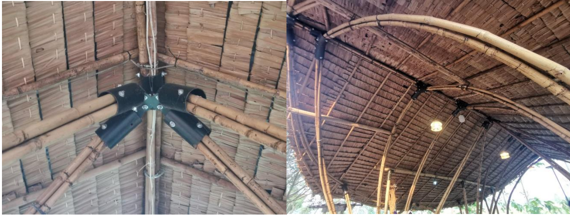
Figure 21. Experiment of pre-fabricated connectors at roof ridges for fast installation.
