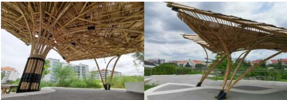
Fig.17. Experiment of Bamboo pavilion using connectors to put together bamboo splits, bundles, splices and at base by Thammasat Bamboo studio.
