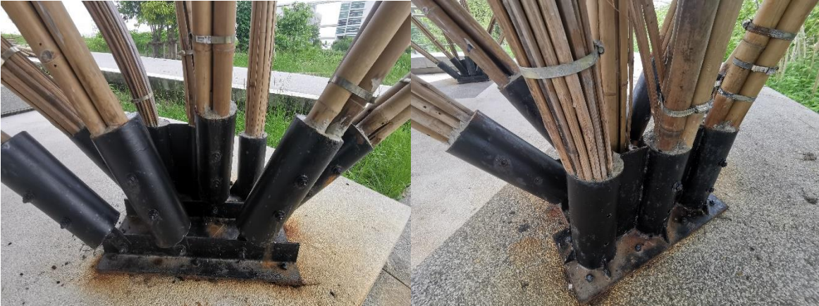
Figure 20. Installation of multiple-members connectors at base foundation
