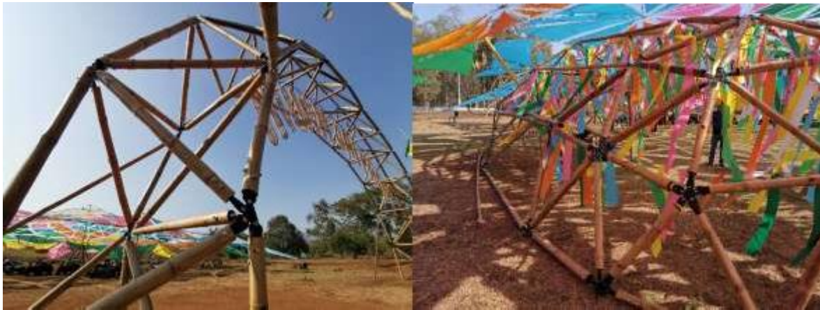
Fig. 15. With flexibility of connecting elements, the designed truss frame can offer variety of design. Creating gateway truss (Left) or Geodesic dome (right) are also possible, by simply putting together with simple tools.
